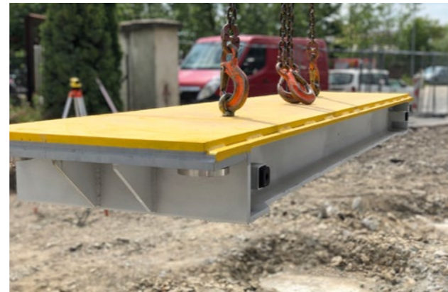
Axle weigh bridge before settling in the frame
